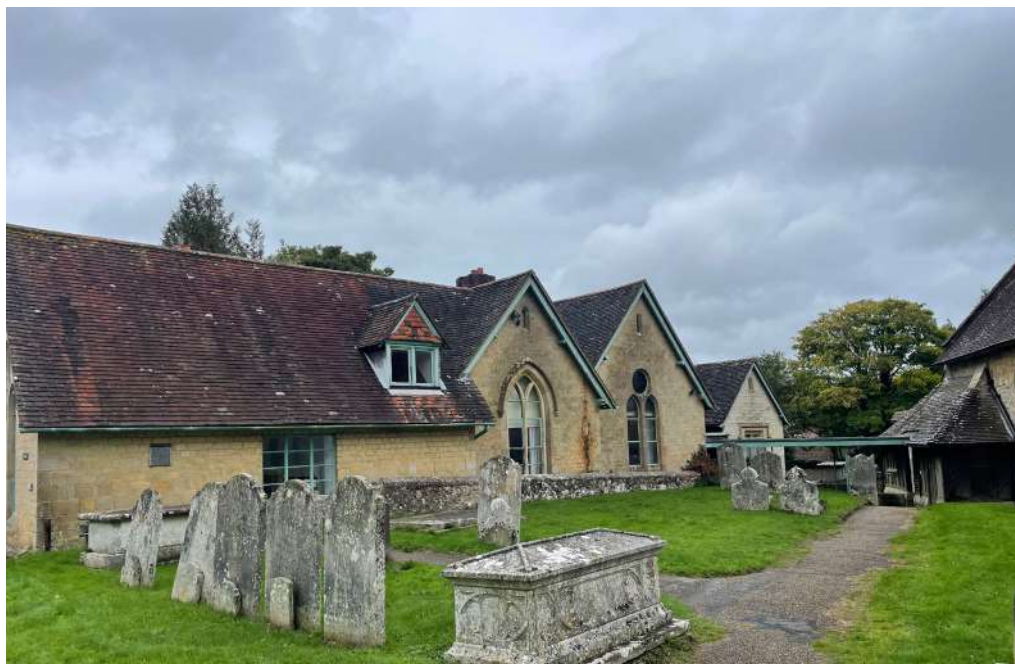
Figure 5.0- View from the west looking at the southwest elevation
