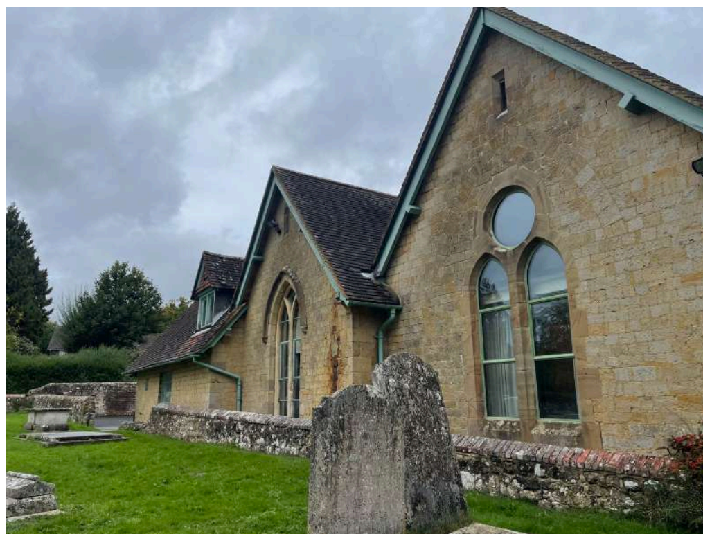
Figure 5.1 - View from east, looking at the southwest elevation
