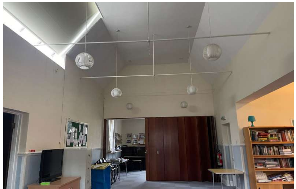
Figure 5.6 - Internal view, looking east. Shows roof light and internal beam, both added in the 1990's.
