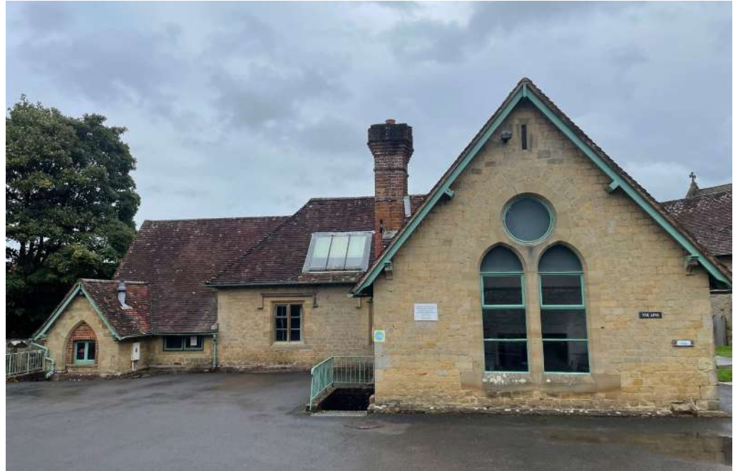
Figure 5.2 - View from the west, looking at the north west elevation
